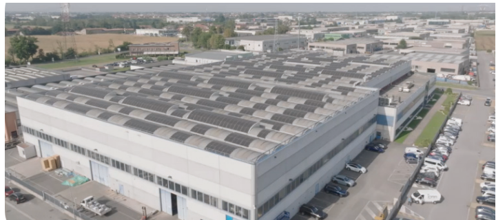
Solar power energy generation and use of electric car
